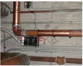
Vulcan unit installed on water main
