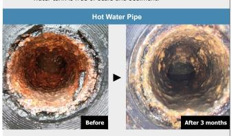
After 3 months the rust in the pipe has lightened and the amount of scale is gradually reducing.
