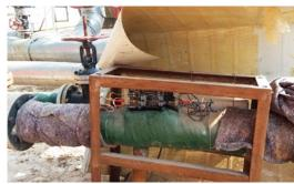
Before installing Vulcan, the rust and pipe insulation were removed, and the impulse bands were winded on the pipe. Then, the outer insulation was put back.
