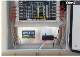
Connect the Vulcan S250 unit with the impulse bands. (Vulcan unit was installed in the outdoor case to prevent from humidity.)
