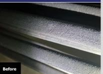
The hard scale between the fins affected the heat transfer efficiency and rusting caused problems with rusty water.
