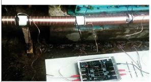
**Picture 1.** Vulcan installation process at the main incoming water line.
