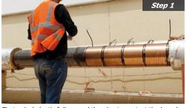
First, wind plastic foil around the pipe to protect the impulse bands against condensation on the pipe.
