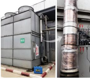
Vulcan S25 was installed at the water inlet of the cooling tower.
