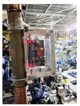
Vulcan S25 is installed on the main pipeline of the circulating water system for the production robots.
