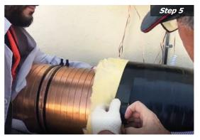
To finish, install an insulation protection to cover the impulse bands completely against the elements.
