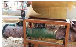
Before installing Vulcan, the rust and pipe insulation were removed, and the impulse bands were winded on the pipe. Then, the outer insulation was put back.
