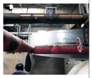
Vulcan S25 installed on DN80 copper pipe.
