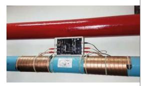
Anti-Scale System Vulcan S25 installed
