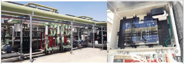
Vulcan S250 outdoor installation: on the roof, with the sun most of the year. The temperature at this time was 38 - 40 °C. In winter, it is rainy and the wrap should be sealed to IP-68. Vulcan impulse bands were well wrapped and the Vulcan unit was in the outdoor box.
