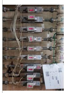
There are 9 secondary small pipes with water meters. These meters were installed to make sure a stable flow rate. If the flow rate goes down, it would cause a problem of the induction hardening machine. Therefore, the pipes had to be cleaned manually every 2-3 months.
