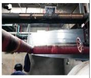
Vulcan S25 installed on DN80 copper pipe.
