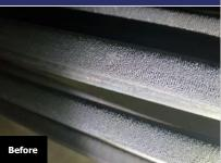
The hard scale between the fins affected the heat transfer efficiency and rusting caused problems with rusty water.
