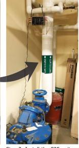
Step 2: Install the S25 unit on the water main and wrap the protection layer
