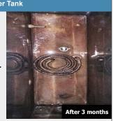
After 3 months scale is no longer forming and the hot water tank is free of scale and sediment.
