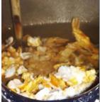
Pictures 2 & 3. Scale previously coating the heating element and reservoir sump. (Picture taken from one of the rooms at IBMA hotel)
