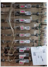
There are 9 secondary small pipes with water meters. These meters were installed to make sure a stable flow rate. If the flow rate goes down, it would cause a problem of the induction hardening machine. Therefore, the pipes had to be cleaned manually every 2-3 months.
