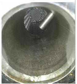
After 3 months – with Vulcan treatment. Up to now the installed pipeline needed no cleaning.
