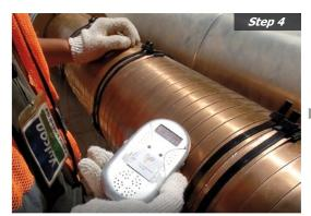
Check the functionality of Vulcan with a impulse detector.
