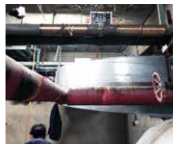
Vulcan S25安装在DN80铜管上
