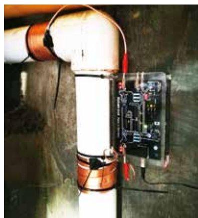
Vulcan S10安装在总出水管道上
