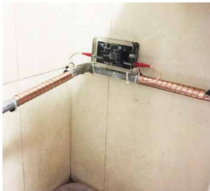
Vulcan 3000安装在学生宿舍里较小的管道
