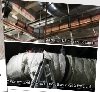
Step 2: Pipe wrapped insulation cotton, then install X-Pro 1 unit!
