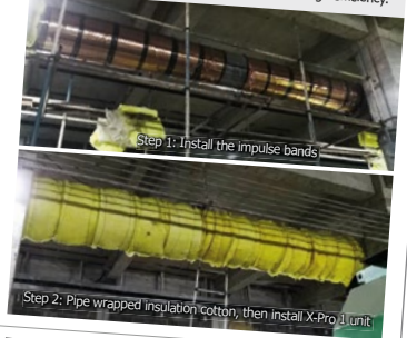
Step 1: Install the impulse bands
