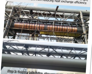
Step 2: Outdoor installation, pipe wrapped insulation cotton, X-Pro 2 unit into the protective box
