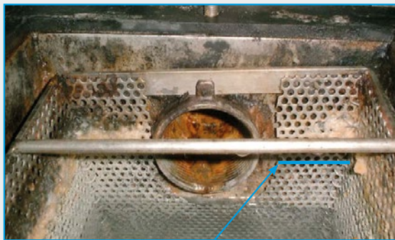
Usual level of standing water.
