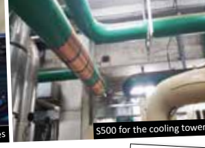
V5000 for the process water pipes
