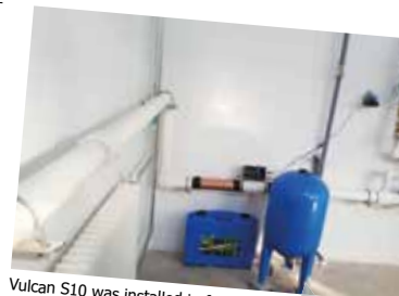
Vulcan S10 was installed in front of the water heater.
