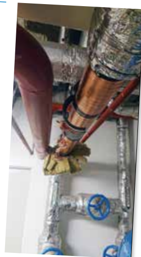
Vulcan S50 was installed on the main inlet of Building A.
