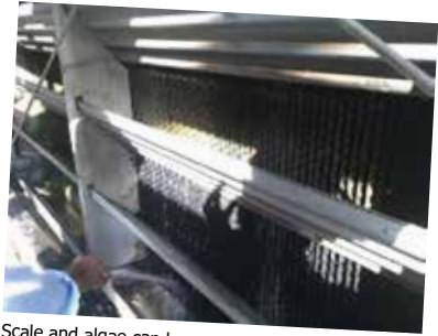
Scale and algae can be removed easily by a water gun.
