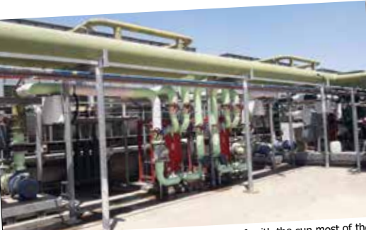
Vulcan S250 outdoor installation: on the roof, with the sun most of the year. The temperature at this time was 38 - 40 °C. In winter, it is rainy and the wrap should be sealed to IP-68. Vulcan impulse bands were well wrapped and the Vulcan unit was in the outdoor box.
