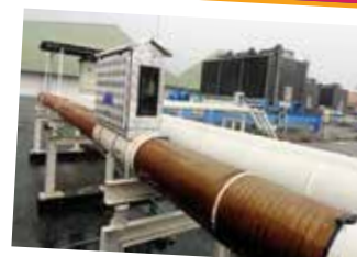
Vulcan S500 was located inside aluminum box and installed on a cooling tower main pipe.
