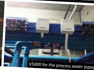
Impulse bands covered by pipe insulation
