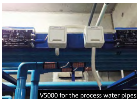
Impulse bands covered by pipe insulation
