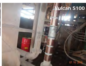
Heat exchanger after 2 months Vulcan installation
