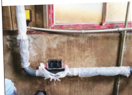
Vulcan S100 was installed in the sewage room to treat the sludge dewatering machine.
