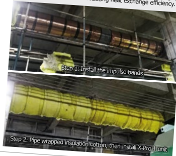
Step 1: Install the impulse bands
