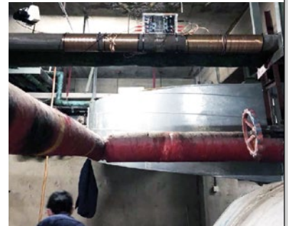
Vulcan S25 installed on DN80 copper pipe.
