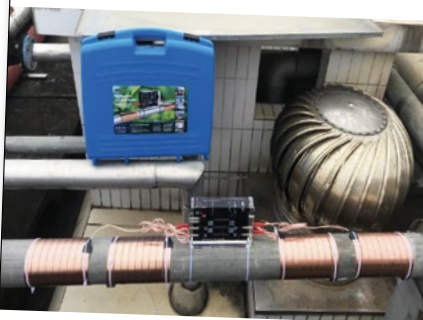
Vulcan S25 was installed on the main water pipe of the guest room Building B.
