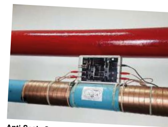
Anti-Scale System Vulcan S25 installed
