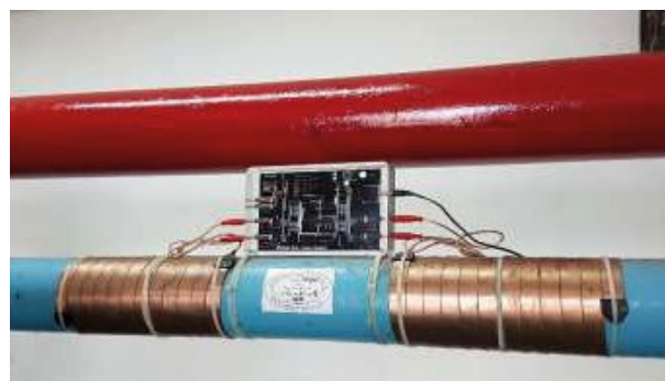
Anti-Scale System Vulcan S25 installed
