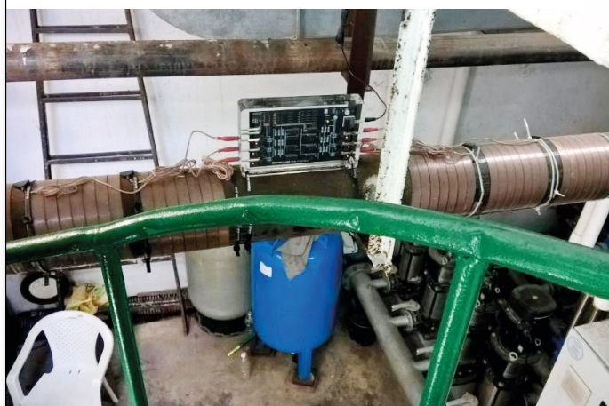
Two Vulcan S100 were installed.
