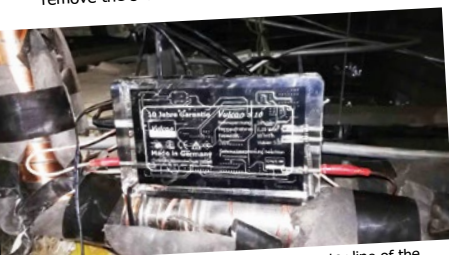
Vulcan S10 was installed on the main water line of the Chinese kitchen.
