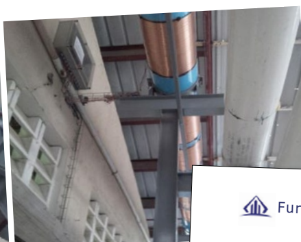
Vulcan S500 cable windings
