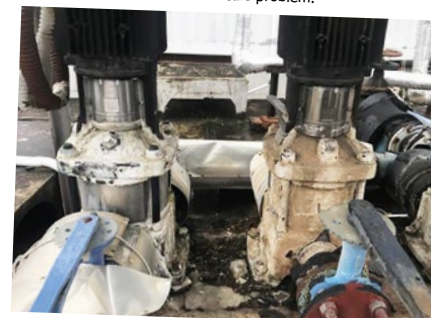
On the left is the pipe (without scale) after Vulcan S25 was installed for 2 months; on the right is the pipe without any water treatment.
