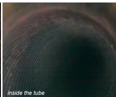
Chiller #3 Condenser Ø 67 cm, tube Ø 7/8", length: 418 cm
