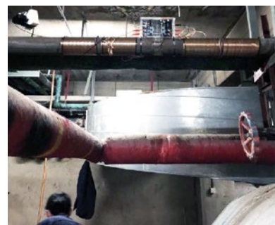
Vulcan S25安装在DN80铜管上
