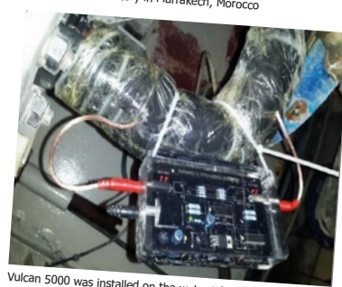
Vulcan 5000 was installed on the water inlet of the water recycling room.
