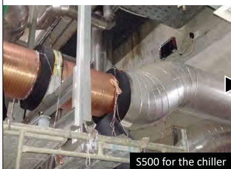
Impulse bands covered by pipe insulation
