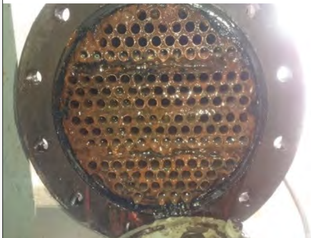
Heat exchanger before Vulcan installation
