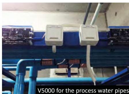
Impulse bands covered by pipe insulation
