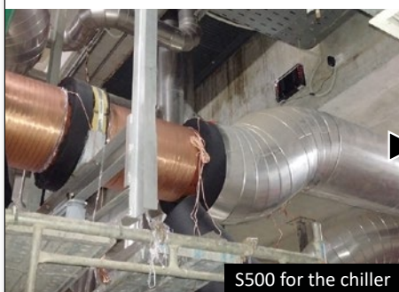
Impulse bands covered by pipe insulation
