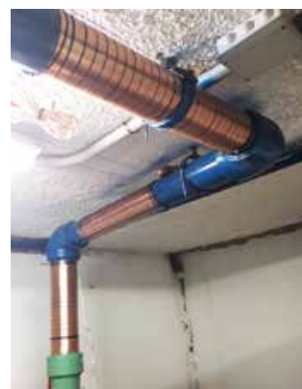
Step 1: Install the impulse bands
