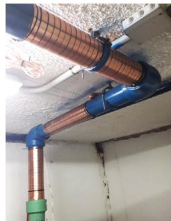
Step 1: Install the impulse bands
