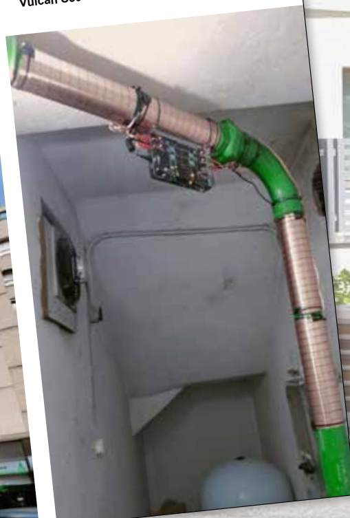
Vulcan S50 Main cold water line with Ø 76 mm
