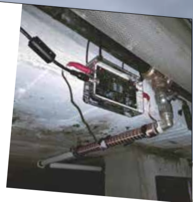
Vulcan 3000 Water deposit line with Ø 25mm
