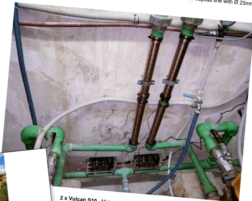
Vulcan 3000 Water deposit line with Ø 25mm
