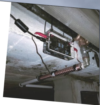
Vulcan 3000 Water deposit line with Ø 25mm
