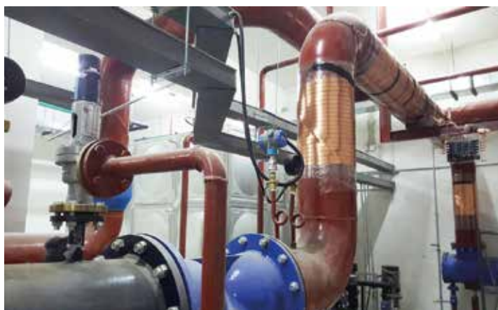
Vulcan S350 was installed in the heating system in the high zone of the heat exchange station.
