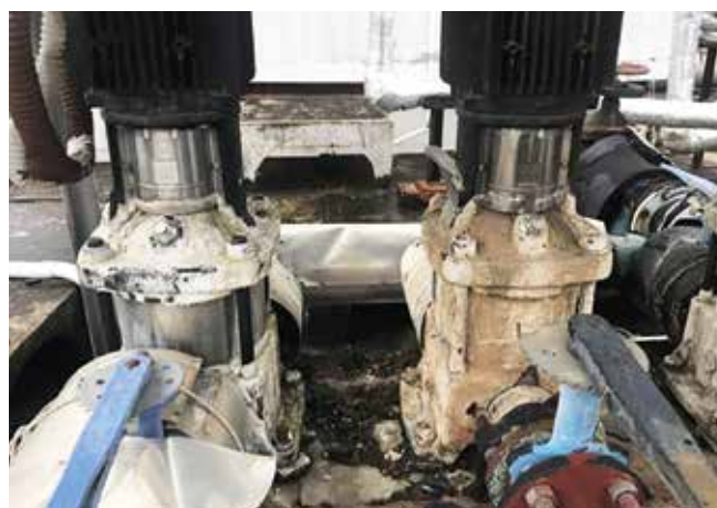
On the left is the pipe (without scale) after Vulcan S25 was installed for 2 months; on the right is the pipe without any water treatment.
