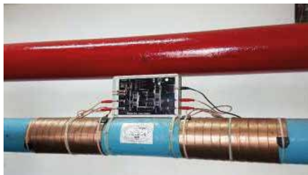
Anti-Scale System Vulcan S25 installed
