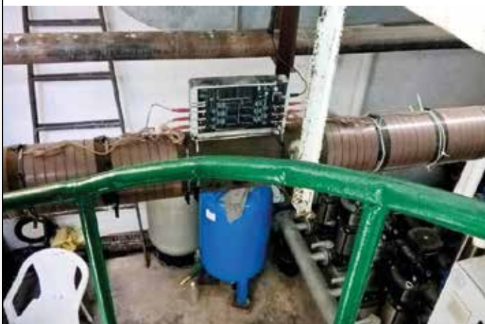
Two Vulcan S100 were installed.
