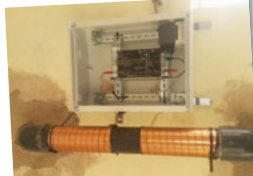
Vulcan S10 was installed in the water main to treat 6 cooling systems in 3 chicken farms.
