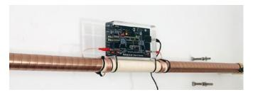
The Vulcan S10 system is installed in the main entrance pipe to the hotel complex for protection and prevention of limescale deposits.
