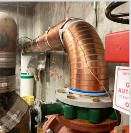
Vulcan S150 impulse bands were installed on the 8-inch water inlet.
