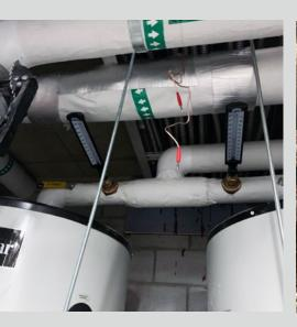
Vulcan S10 was installed on the hot water recirculation on the 27th floor. The impulse bands were covered to prevent condensation before the Vulcan unit was installed.
