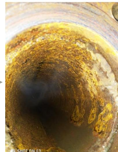
After installing Vulcan for 3 months, the scale has been significantly reduced.
