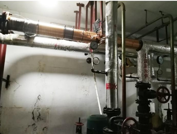
The hot spring water pipeline is far away from the villa, so the water has to be pumped. Vulcan S150 was installed on the delivery pipe.
