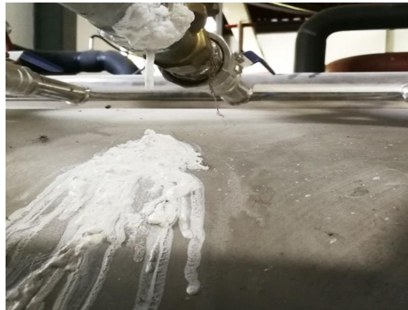
Hot spring water flows out of the pipe joint, it builds up stalactite-like scales over time.
