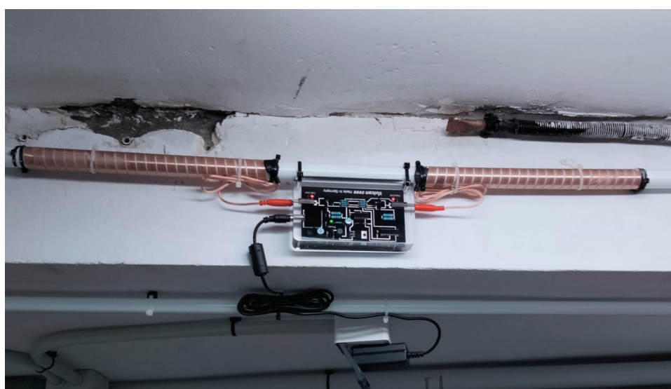
Vulcan 5000 at coldwater main pipe
