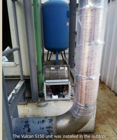
The Vulcan S150 unit was installed in the outdoor case and the impulse bands were covered by the plastic foil against humidity.
