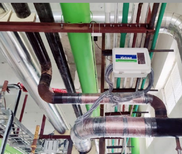
S250 for the extruder chilled water line
