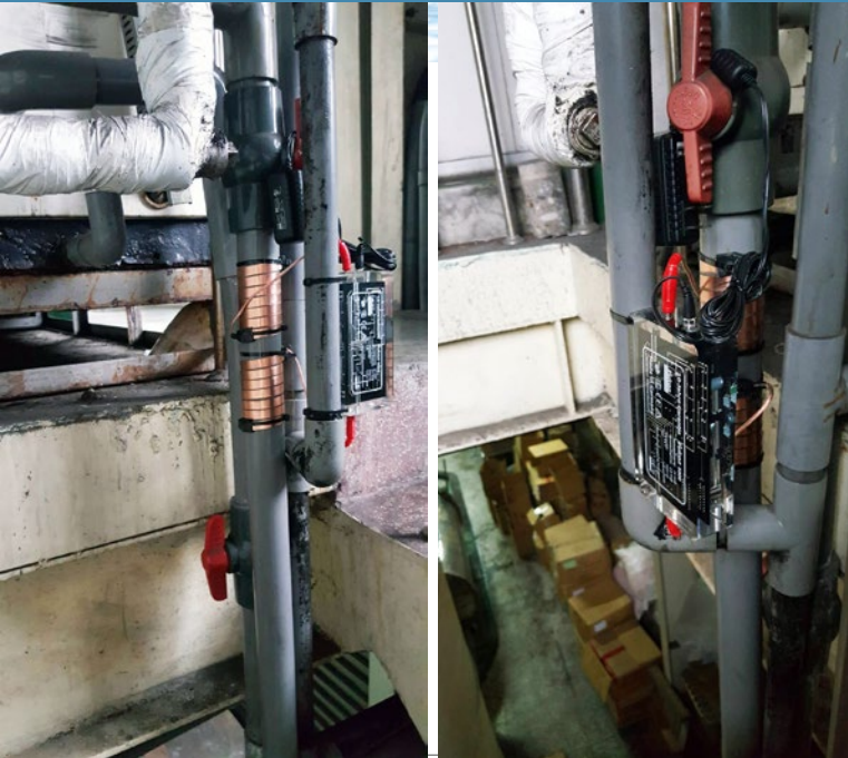
Vulcan 5000 installed on the 2" circulating water pipe
