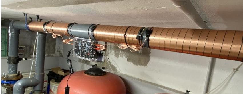
**Vulcan S50** in the swimming pool water circuit N°1 with  $\varnothing$  90 mm
