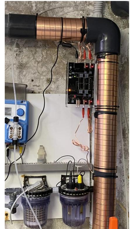
**Vulcan S25** in the swimming pool water circuit N°2 with  $\varnothing$  90 mm
