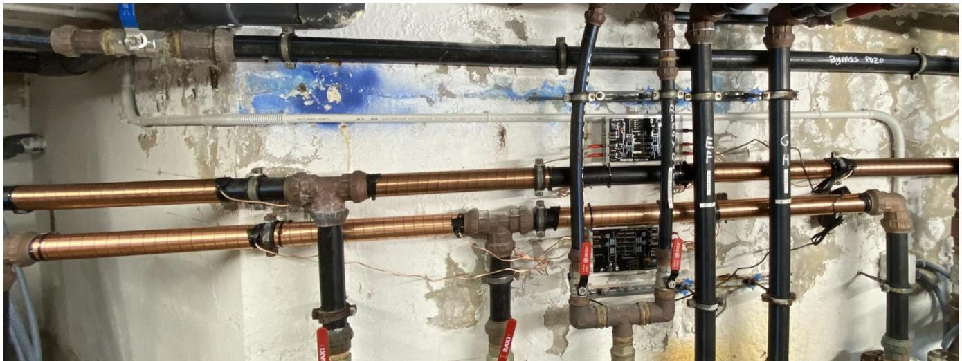
**Vulcan S25** 2 x at the cold water pipe with  $\varnothing$  50 mm for 48 apartments
