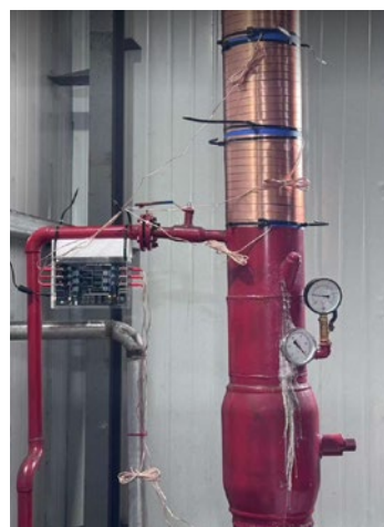
Vulcan S150 for the supply pipeline of the heating boiler
