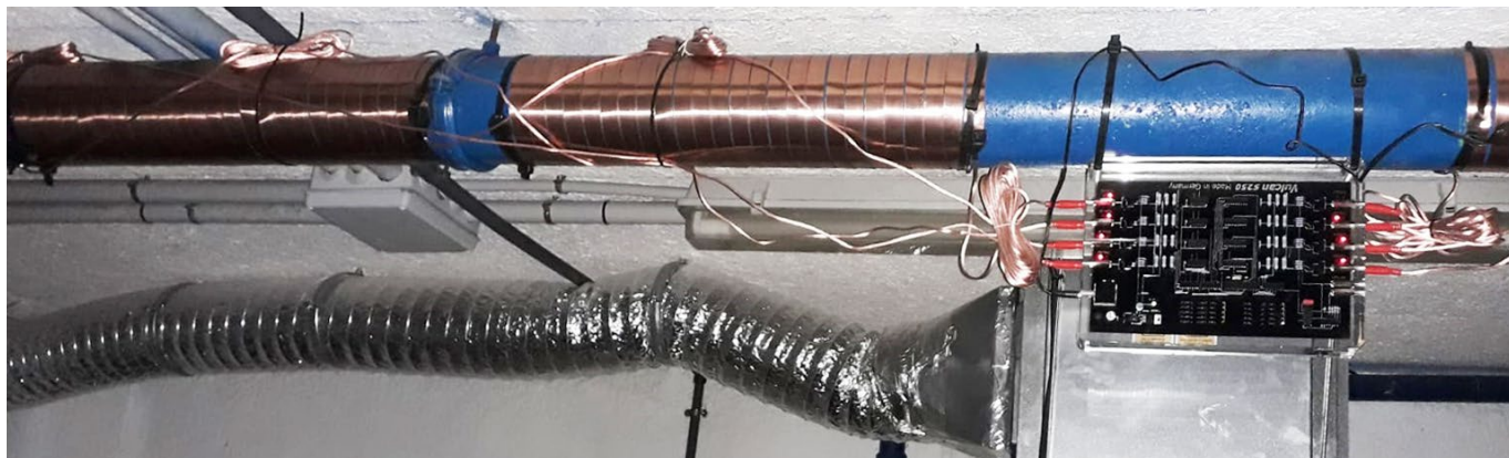
第2步: 将Vulcan S250安装在主水管上
