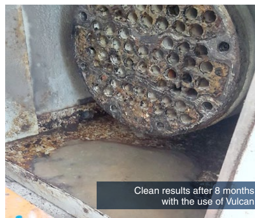
Limescale deposits after 3 months without the use of Vulcan
